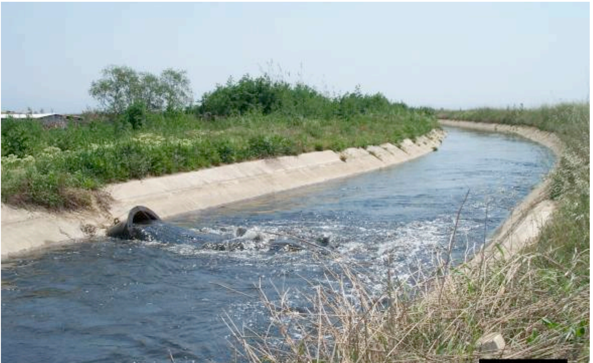
Irrigation canal and mixing point of Thessaloniki's WWTP effluent with the Axios river water
